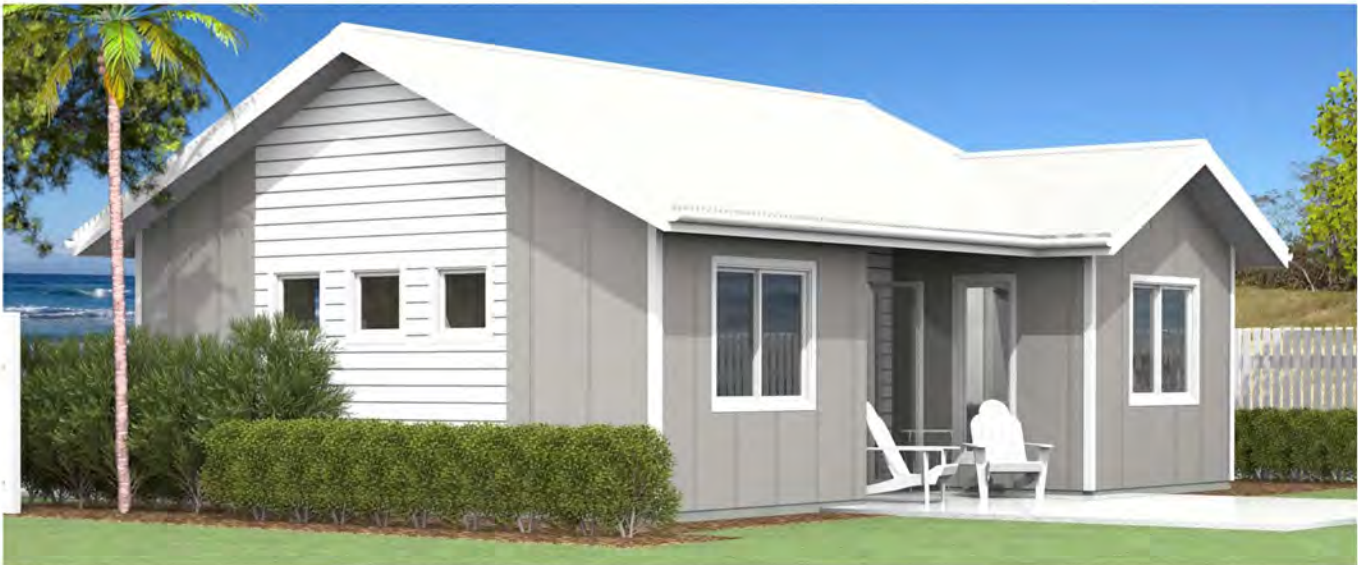
2.6 m High Ground Floor Ceilings
